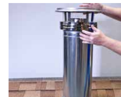
15. Press chimney cap into the last section of pipe. To clean remove the (4) screws and brush the inner sleeve.
