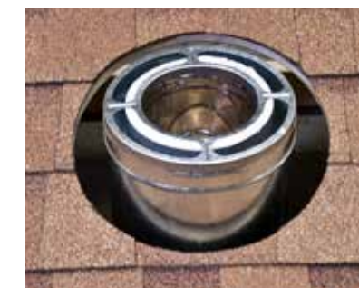
10. Complete the chimney installation above the roof by adding more chimney sections. Make sure the chimney is plumb.
