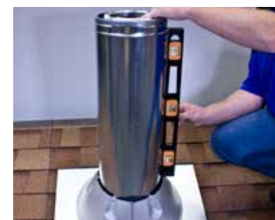
12. Add more chimney sections until chimney is at least 3 ft above roof, and at least 2 ft above any part of your house within 10 ft.
