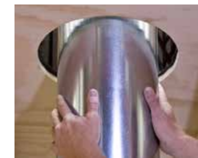
9. Hole in roof must provide at least a 2" clearance all around the chimney. Add more chimney sections, and twist to lock.
