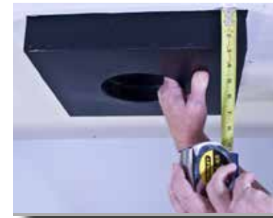
2. Slide the chimney support box into the framed opening from below, and level it. At least 2" of the box should extend below finished ceiling.
