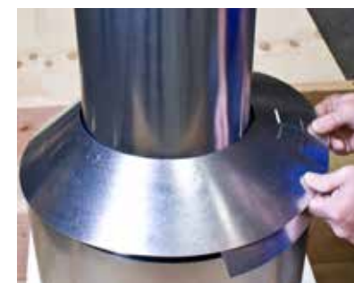
7. Wrap insulation shield collar around chimney. Slide it down to the shield.
