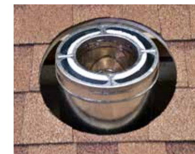
10. Complete the chimney installation above the roof by adding more chimney sections. Make sure the chimney is plumb.
