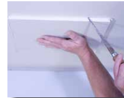
1. Drop a plumb line to center of stove flue collar. Mark center point on ceiling, and cut and frame a 14 1/2" square opening around this center point.
