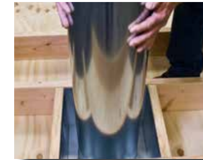
5. Lower the first chimney section over short piece of pipe in the bottom of the support box. Push together and twist to lock.
