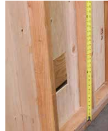
1. Locate appliance and penetration through wall.
