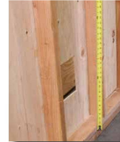
1. Locate appliance and penetration through wall.
