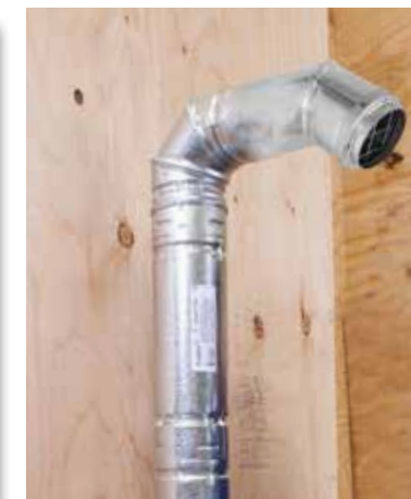
10. Attach horizontal cap to the top elbow.
