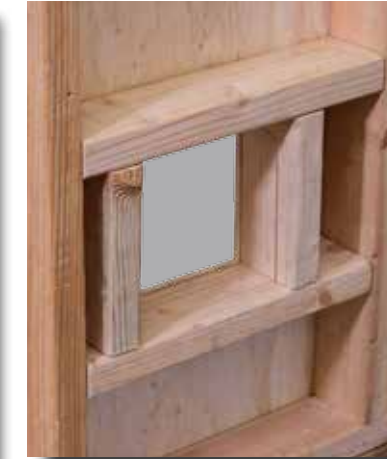
2. Cut and frame wall penetration.
