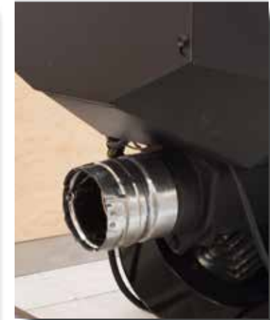
4. Slide appliance adapter onto the appliance outlet and secure with at least one screw.
