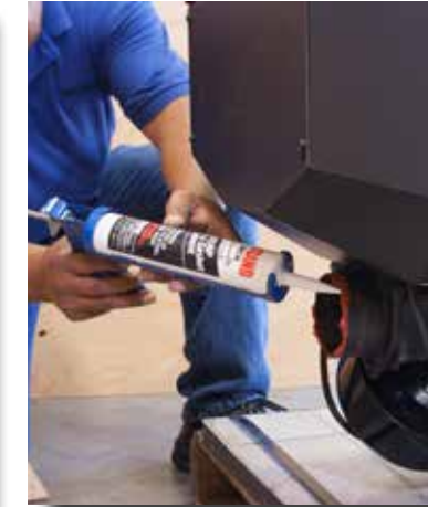
3. Apply high temperature silicone sealant to the appliance outlet.
