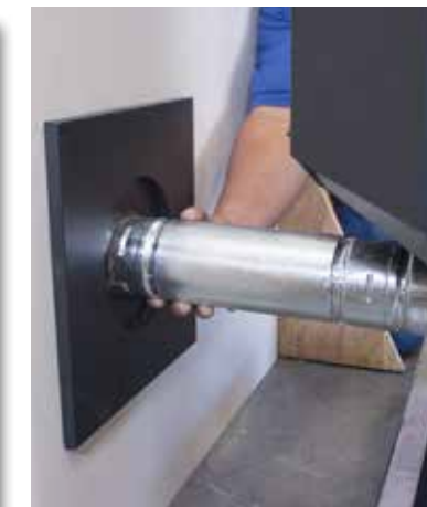
7. Slide pipe through the wall thimble and attach to the appliance adapter on the stove collar.
