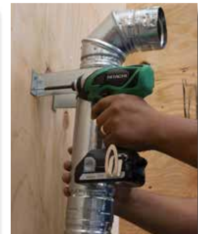
9. Plumb pipe and secure pipe to the wall with wall strap.
