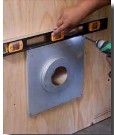
5. Slide outside portion of the wall thimble into the framing. Level and attach to wall.
