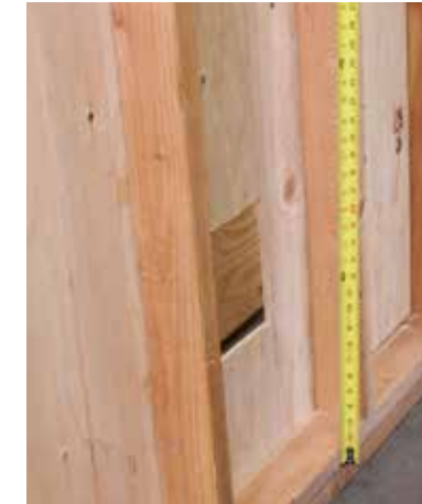
1. Locate appliance and penetration through wall.
