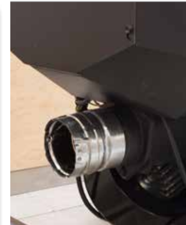
4. Slide appliance adapter onto the appliance outlet and secure with at least one screw.
