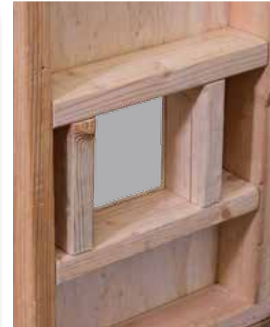
2. Cut and frame wall penetration.
