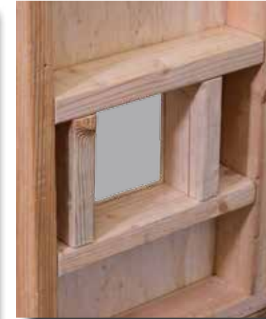
2. Cut and frame wall penetration.
