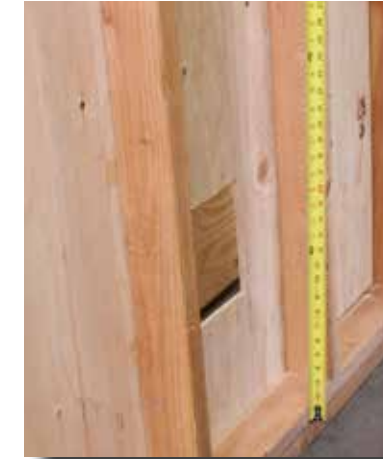
1. Locate appliance and penetration through wall.
