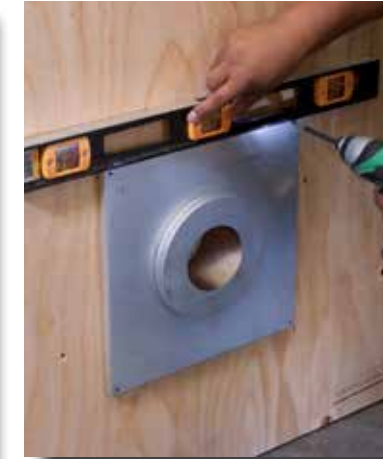
5. Slide outside portion of the wall thimble into the framing. Level and attach to wall.
