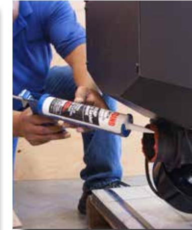
3. Apply high temperature silicone sealant to the appliance outlet.
