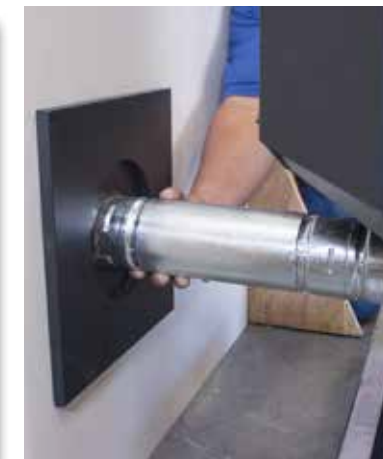
7. Slide pipe through the wall thimble and attach to the appliance adapter on the stove collar.
