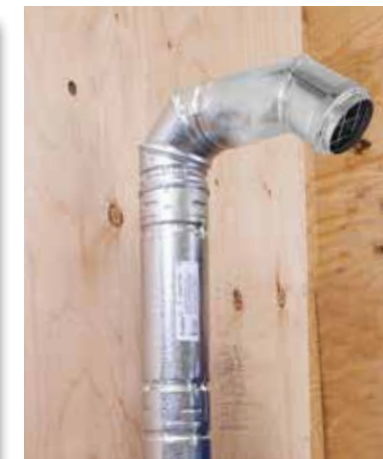
10. Attach horizontal cap to the top elbow.
