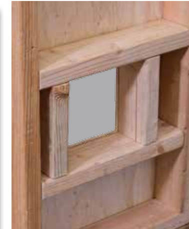
2. Cut and frame wall penetration.
