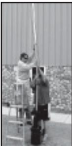
7. Using a ladder and a helper, place the remaining pole sections atop the standing sections.
