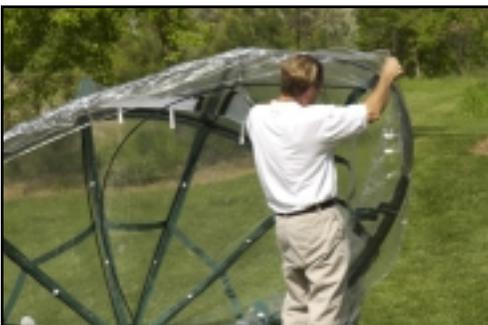
8. Repeat inserting poles in top then bottom pockets and fasten in place as you go.
