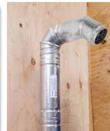
10. Attach horizontal cap to the top elbow.
