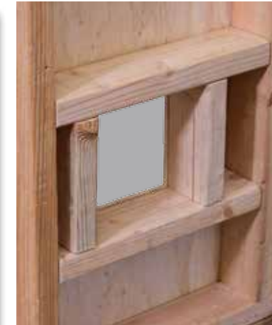
2. Cut and frame wall penetration.
